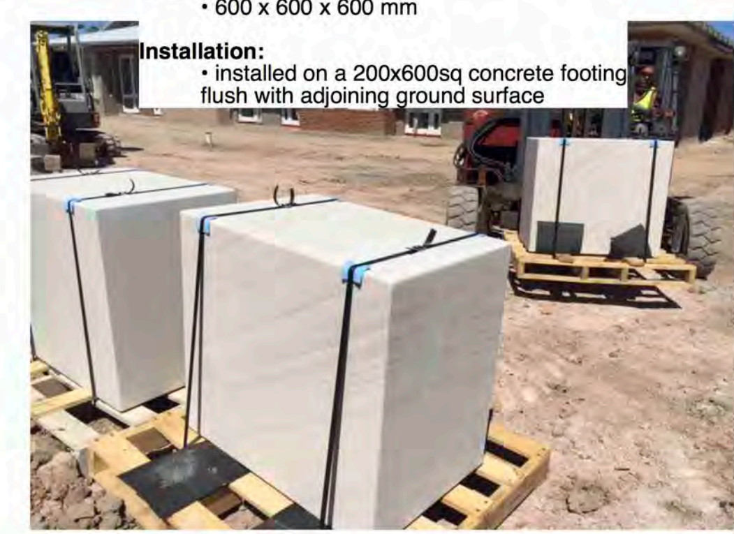
3 SANDSTONE BOLLARDS 1:20@A1
